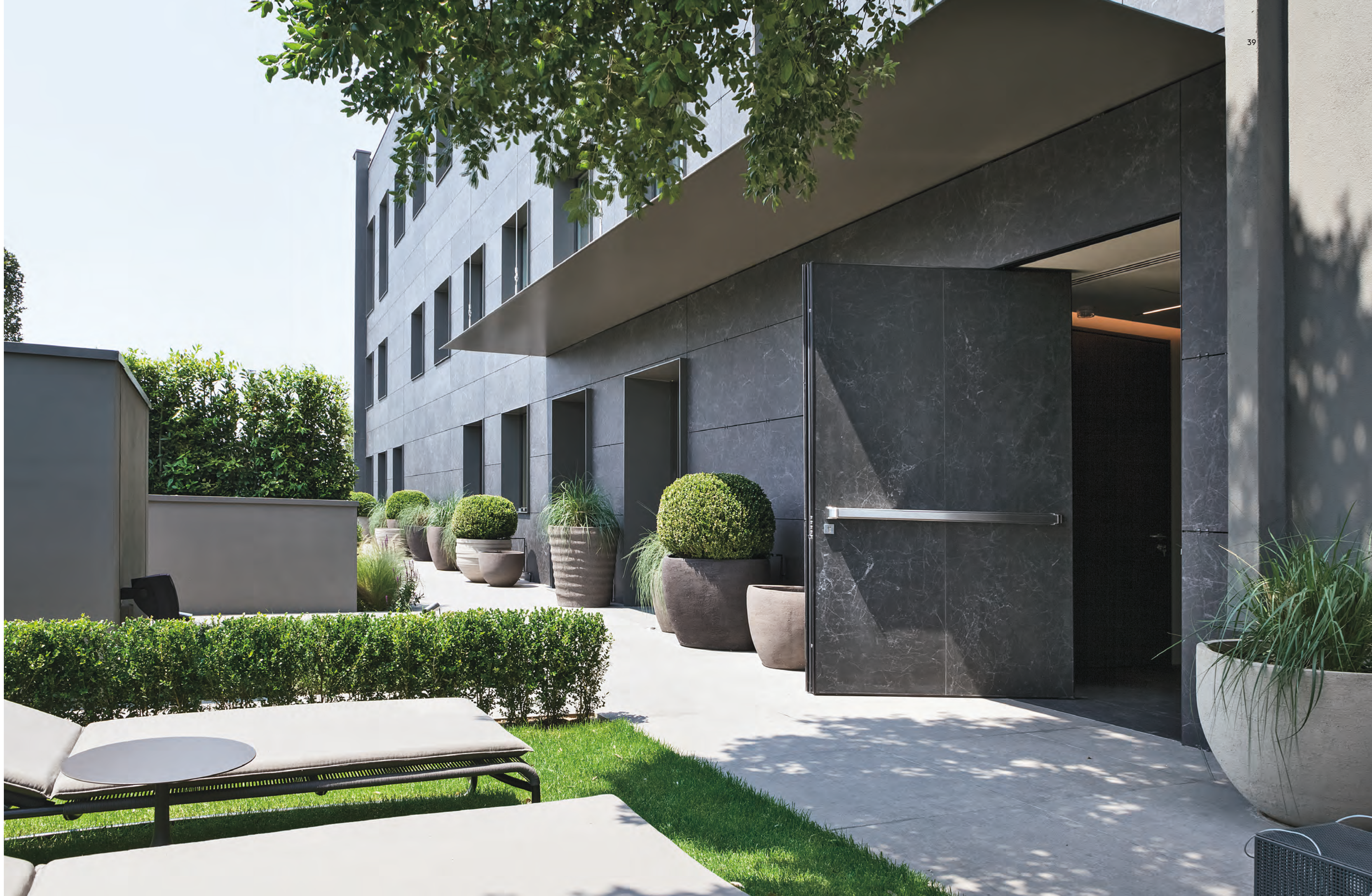
Bergamo, Italy Furniture Showroom Main entrance with Synua door and panic long handle. Laminam customized cladding.
